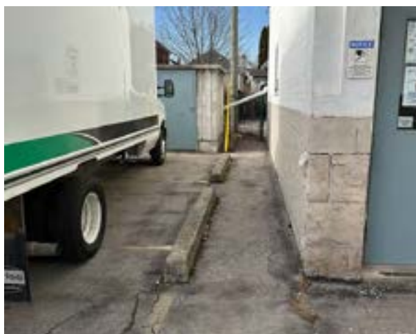
Image 15 Asphalt along building facade
