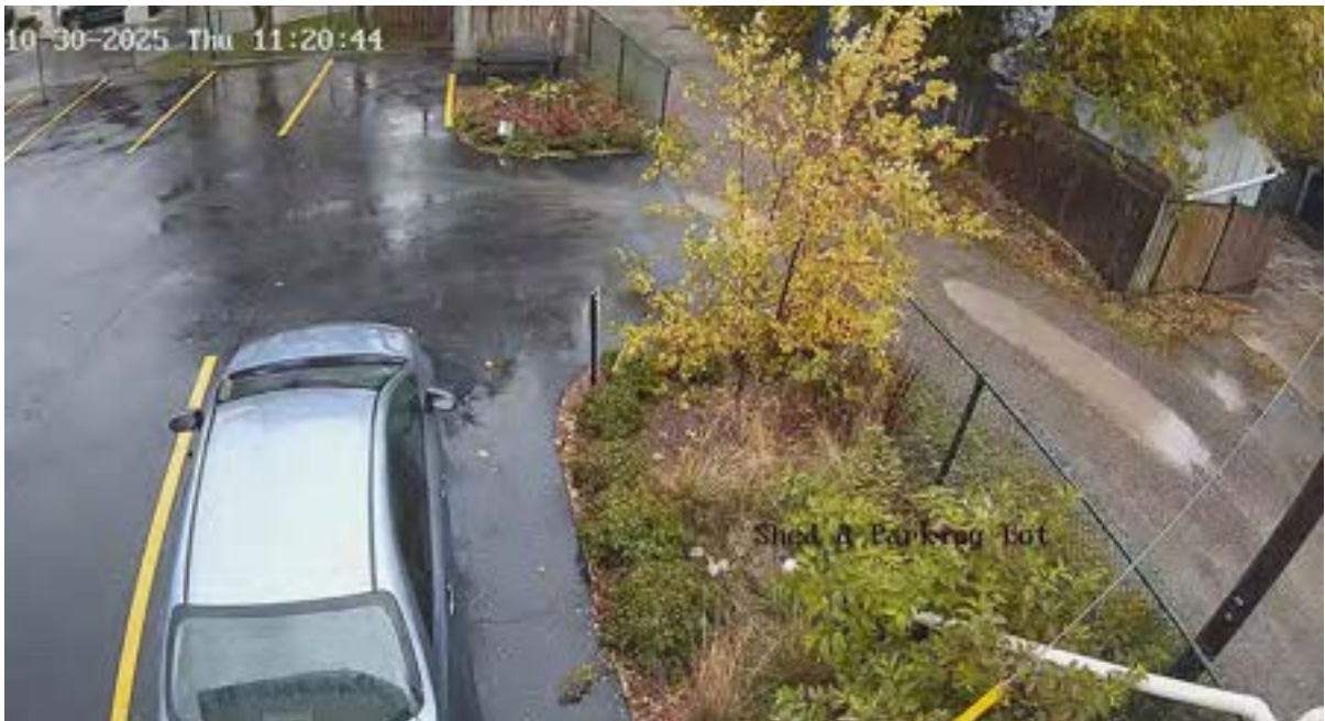
Image 32 Rain Garden October 30, 11:20am No overflow, rainwater from downspout appears to be totally infiltrated
