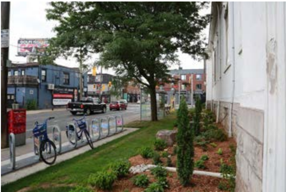
Image 21 New plantings, water slowed at downspout termination
