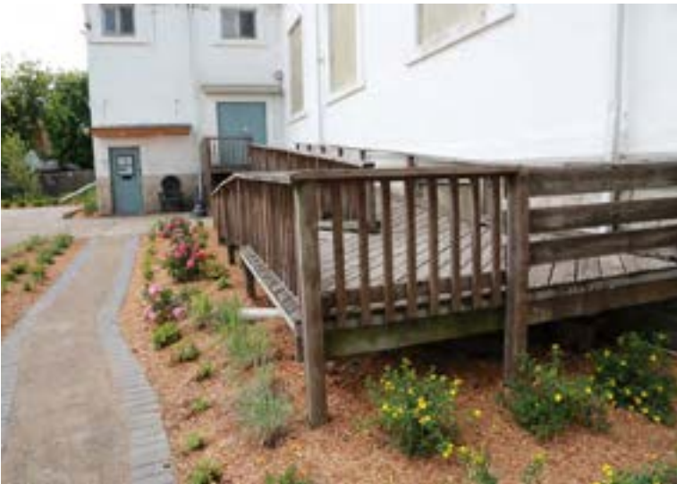
Image 11 Permeable walkway Downspout not yet connected to rain barrel
