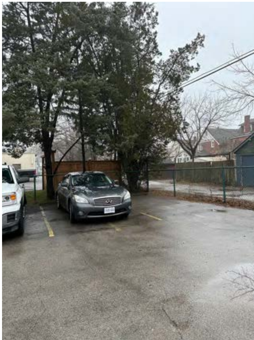
Image 17 Existing asphalt surface
