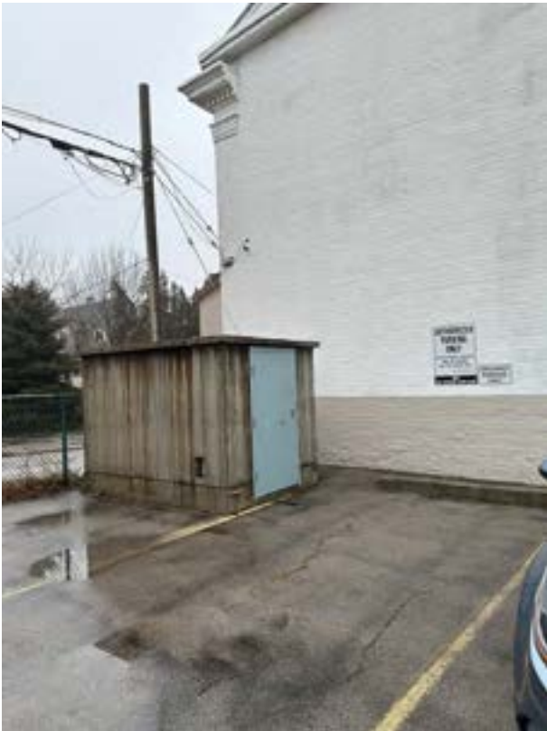
Image 13 Existing location of shed on asphalt
